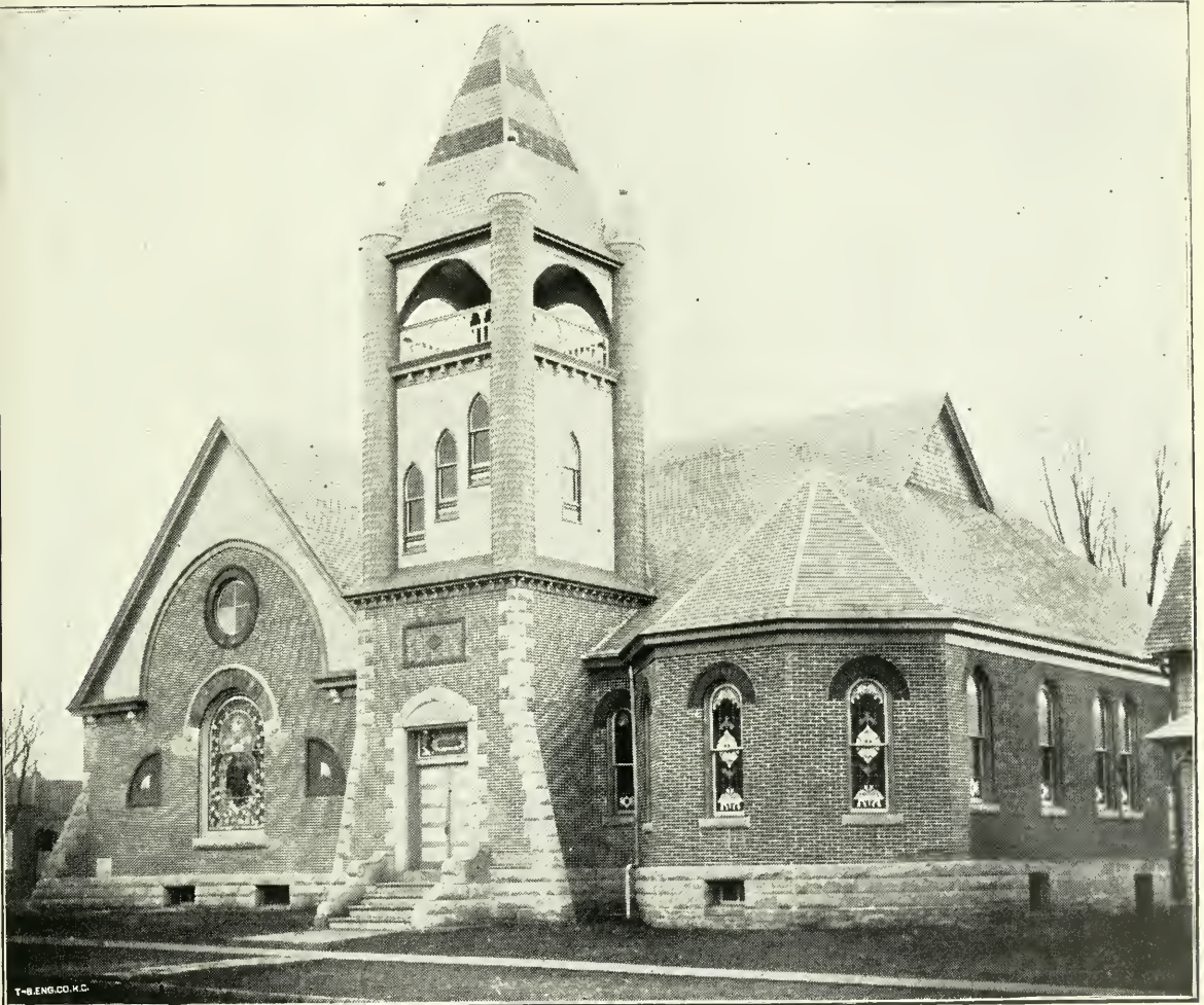
OHIO STREET METHODIST CHURCH, BUTLER, MISSOURI.
